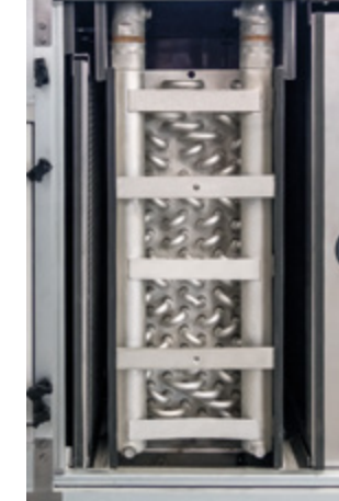
Heat exchanger with sea air resistant coating
