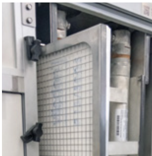
Panel filter with plug-in frame for changing the filter mats
